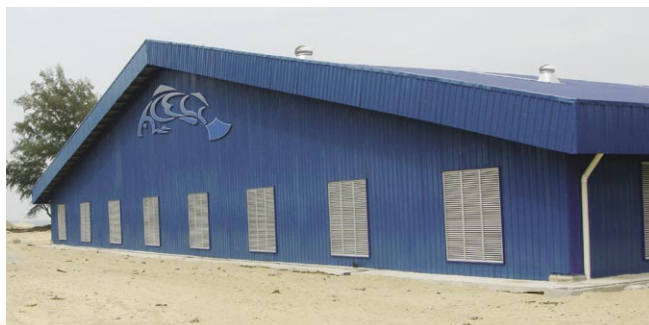
Above: Stage 1 – 2,500m 2 Production Building Now Complete.
