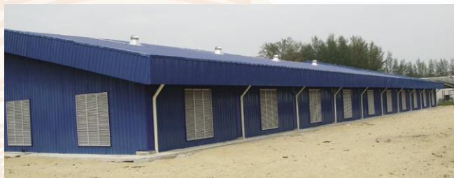
Below: Stage 1 Production Building - Side View.
